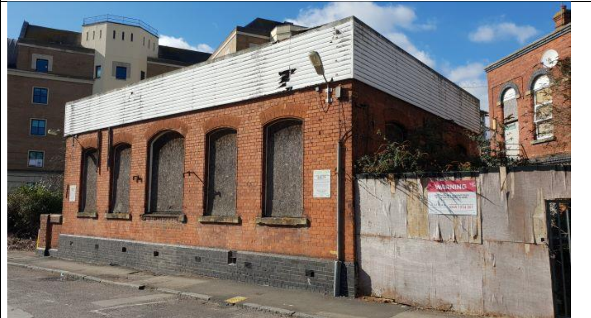
Fig. 11: Gas Governor House. (RBC - April 2022.)
